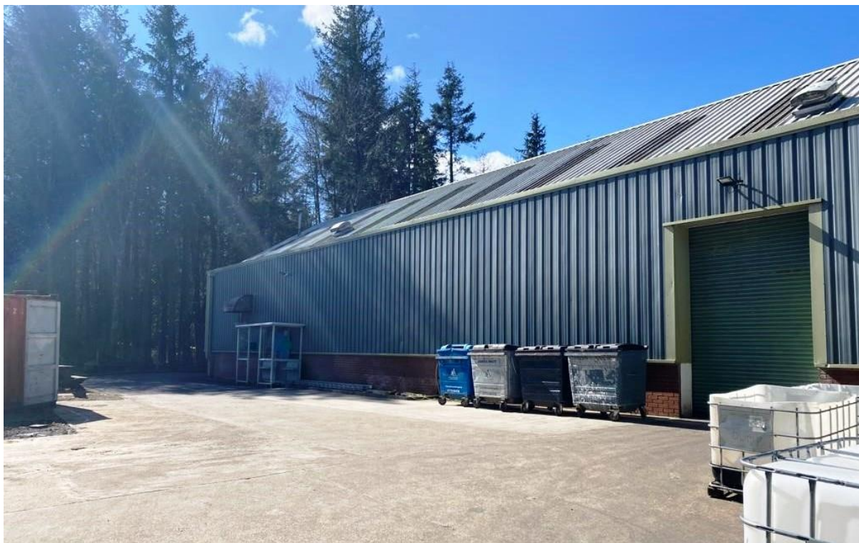
Figure 1 - warehouse suitable for solar PV panel array
